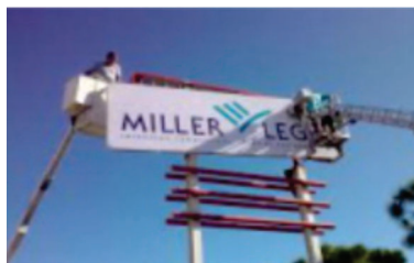
Installing a Flex Face Retrofit to existing cabinet
